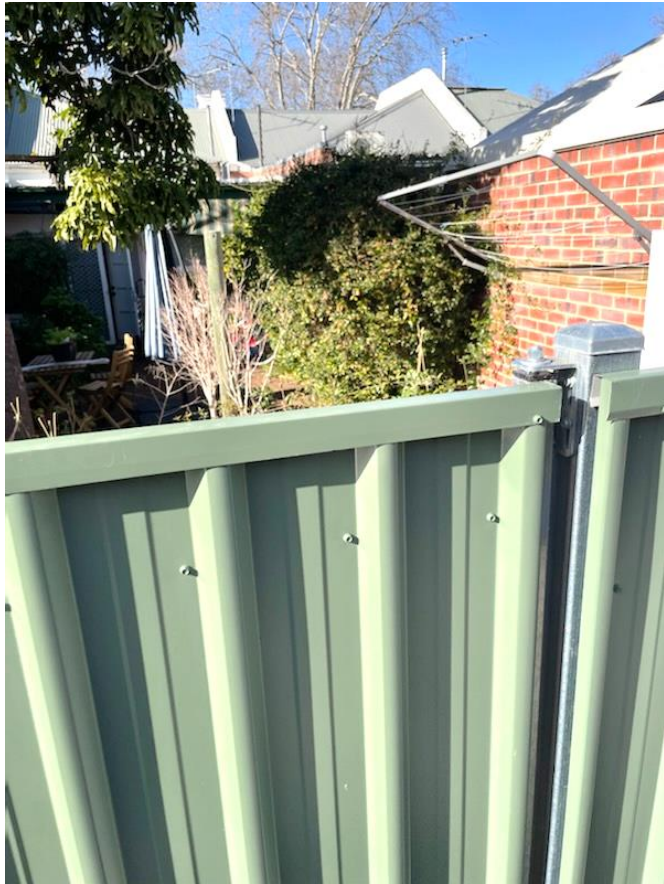
Photo 3.7.7 - Looking south towards subject site and neighbour's garage wall (118 Stanley Street)
